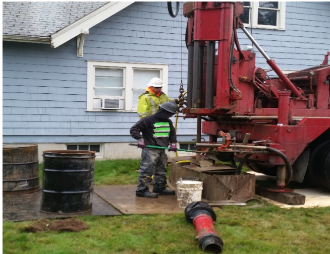
Figure 13- Boring location B-2 overview looking southeast
