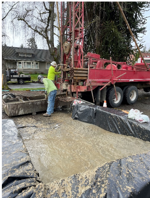
Figure 15- Mud Rotary Drilling operation looking south
