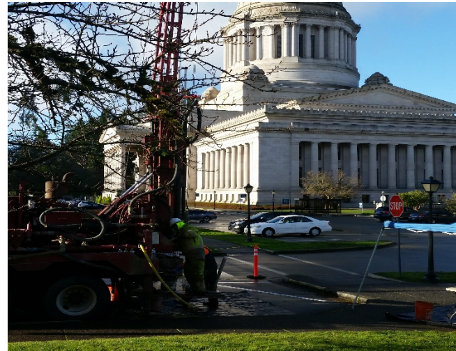
Figure 14- Boring location B-4a overview looking west
