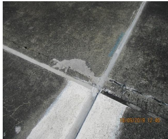
26 - Expansion joint at roof center
