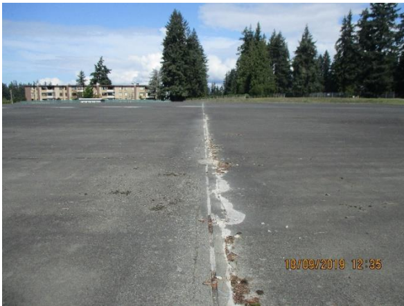
27 - View from south edge of roof, looking north
