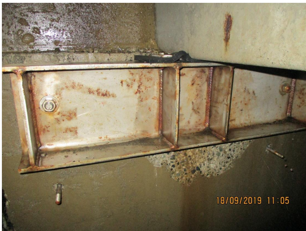
Photo 24 – Previous double-tee support repair near Grid A/B-8
