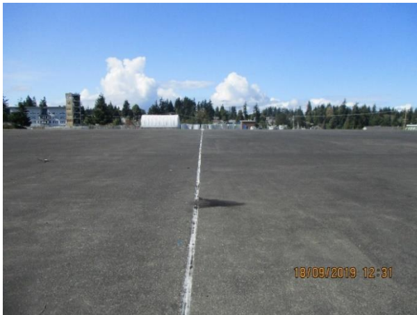
25 - View from center of roof, looking west
