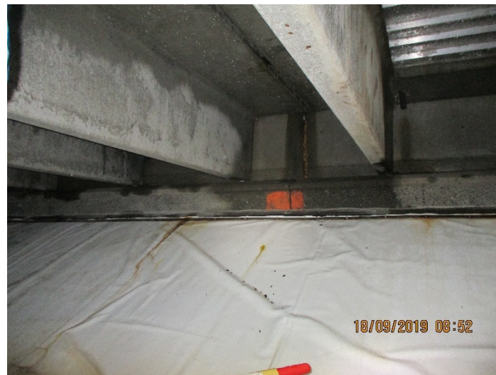
Figure 2 – Existing Hypalon Liner
