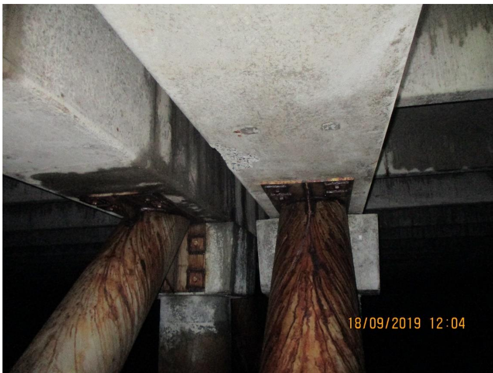
Photo 23 - Standing water at corner crawlspace (typical condition)
