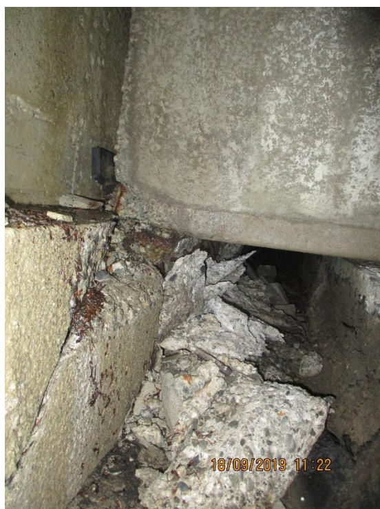
Photo 6 - Concrete girder support at Grid A-8 (opposite side as previous photo)
