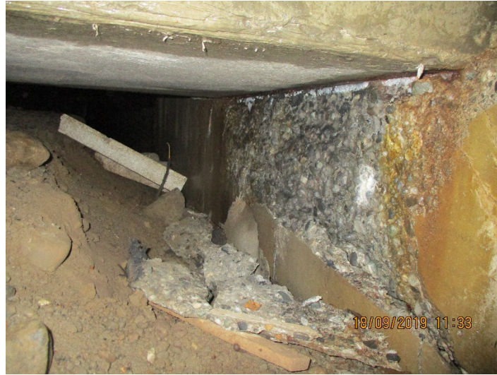
Figure 1 – Typical Girder Support Repair Location
