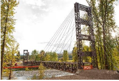
Spring Creek Pedestrian Bridge (Design-Build) Winthrop, WA
