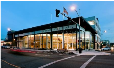
Olympia City Hall (Design-Build) Olympia, WA
