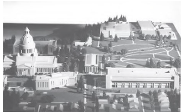
FIGURE 3-5 1974: EXECUTIVE OFFICE BUILDING
