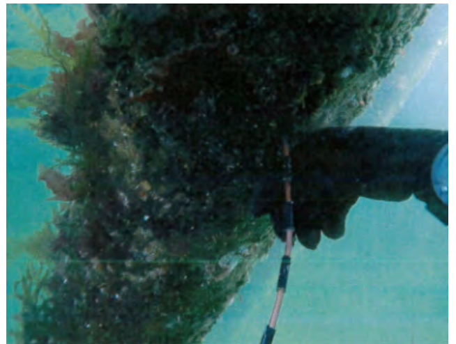
Photo 13: Pile 7.1H marine borer entry (MBE)
