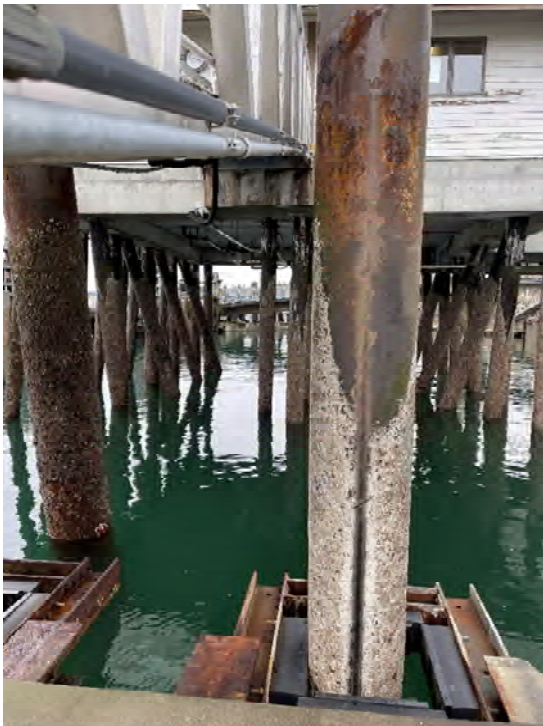
Photo 23: Clearance from pile and loading ramp
