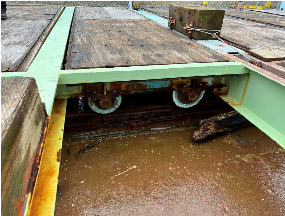
Photo 181: Cradle wheels and decking
