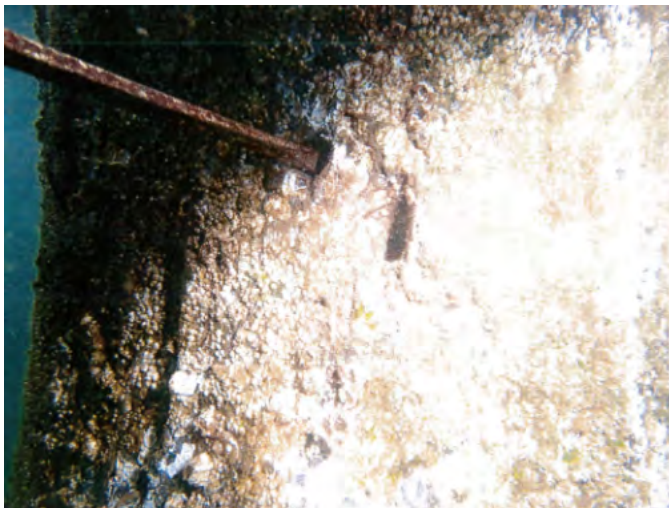
Photo 12: Pile 3B two marine borer entries (MBE)
