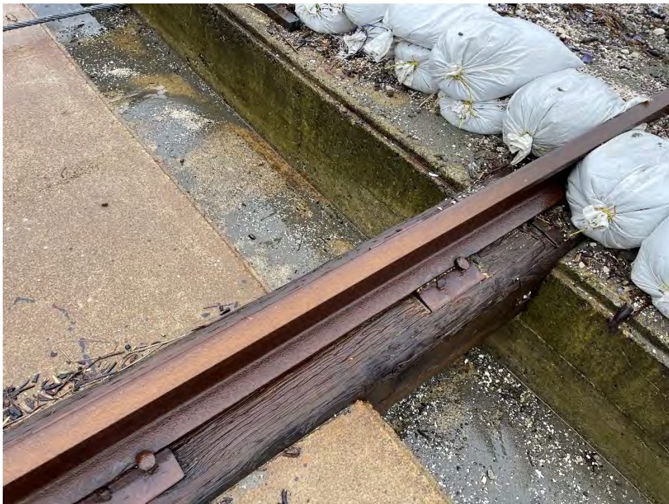
Photo 132: Timber rail and rail North of bulkhead
