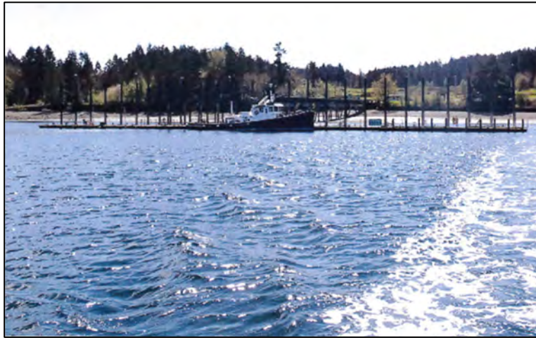
Photo 6: Still Harbor Dock
