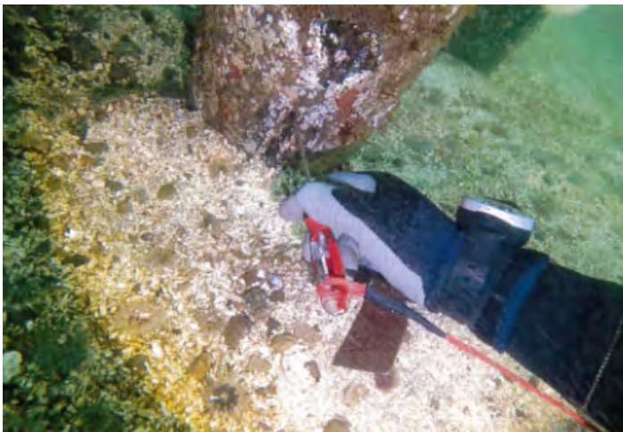
Photo 93: Right wingwall, pile 31 with MBE
