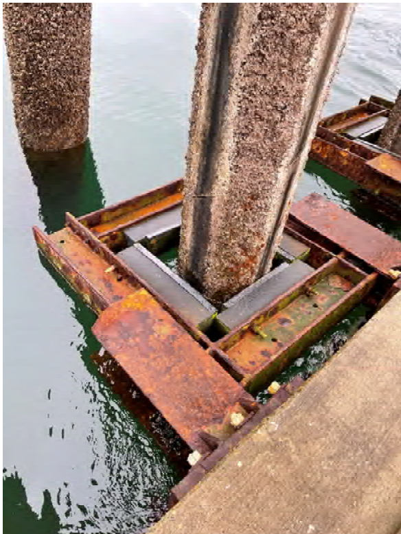
Photo 27: Pile collar with bent angle
