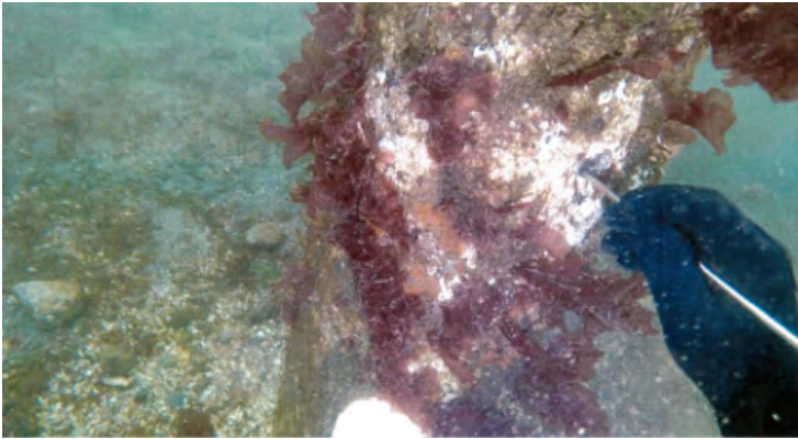
Photo 12: Pile 3B two marine borer entries (MBE)
