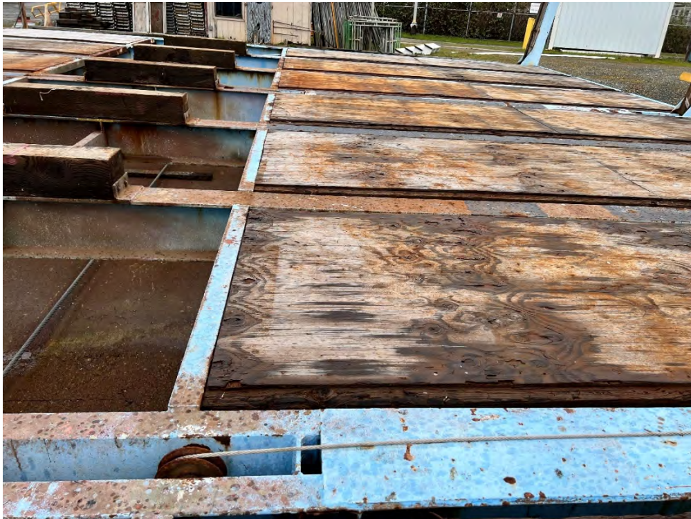
Photo 190: Bilge block pulley
