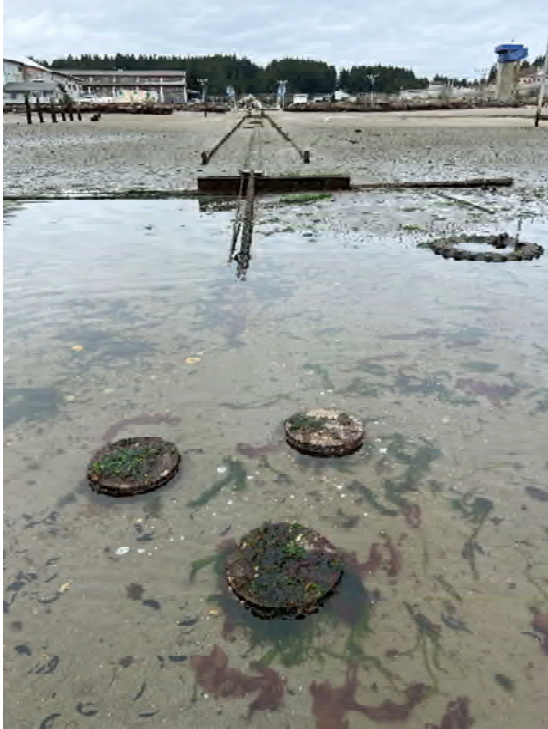
Photo 156: Anchor piles at end of track
