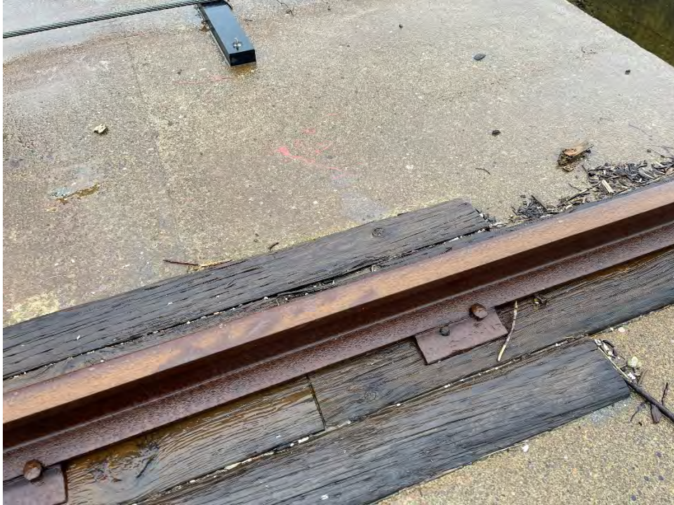
Photo 131: Timber rail and rail North of bulkhead
