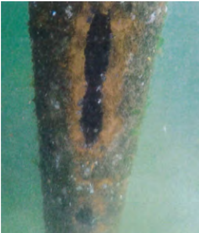
Photo 124: Pile Y, 3" W x 18" H hole and 3" W x 6" H hole from mechanical abrasion
