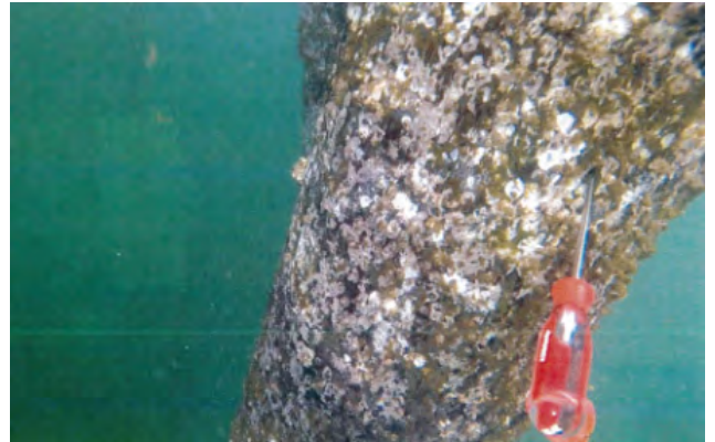
Photo 13: Pile 7.1H marine borer entry (MBE)
