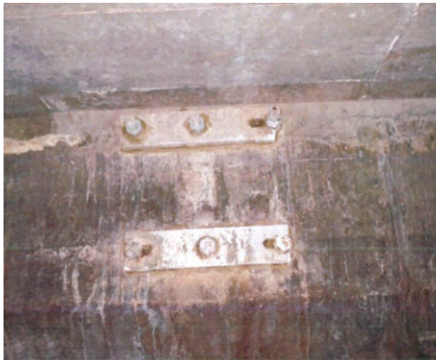
Photo 31: Cell #8 pile collar connections
