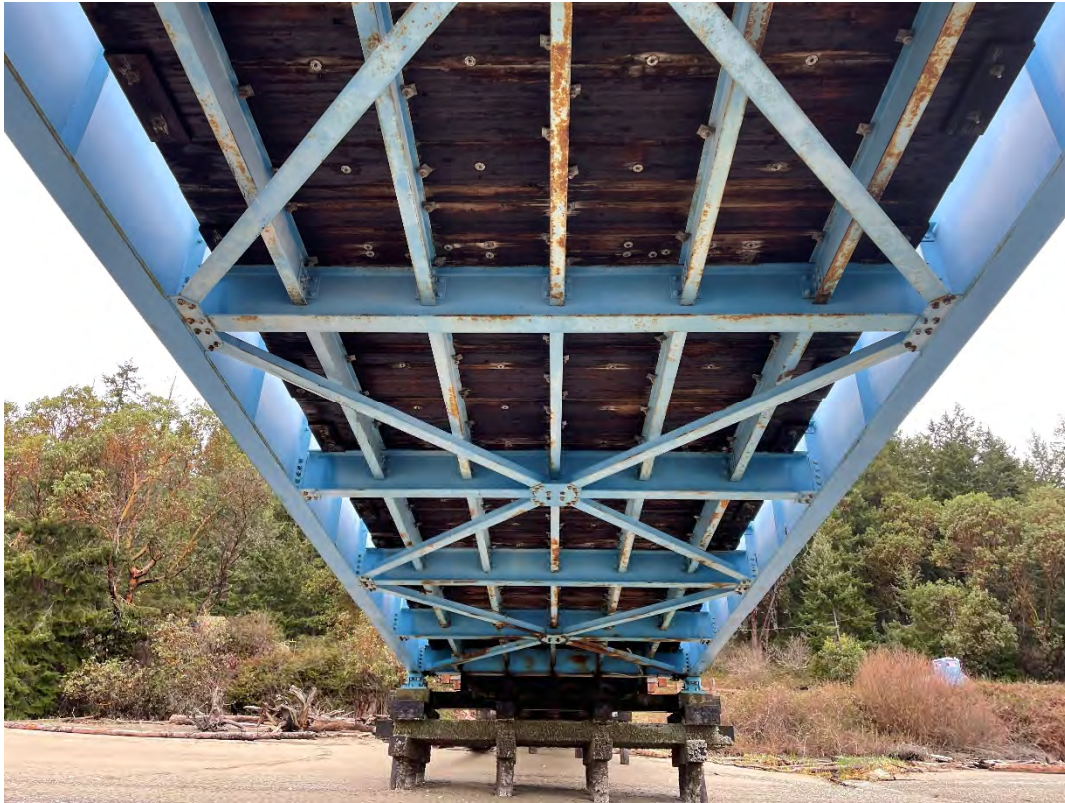
Photo 96: Beneath the trestle
