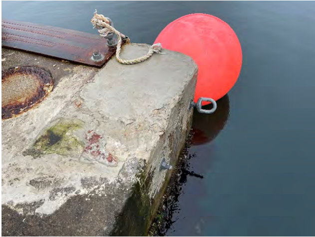
Photo 51: Fender removed and concrete float patched
