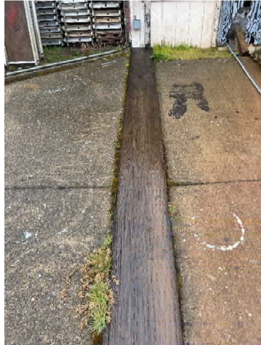
Photo 129: Timber rail beam (B) North of bulkhead
