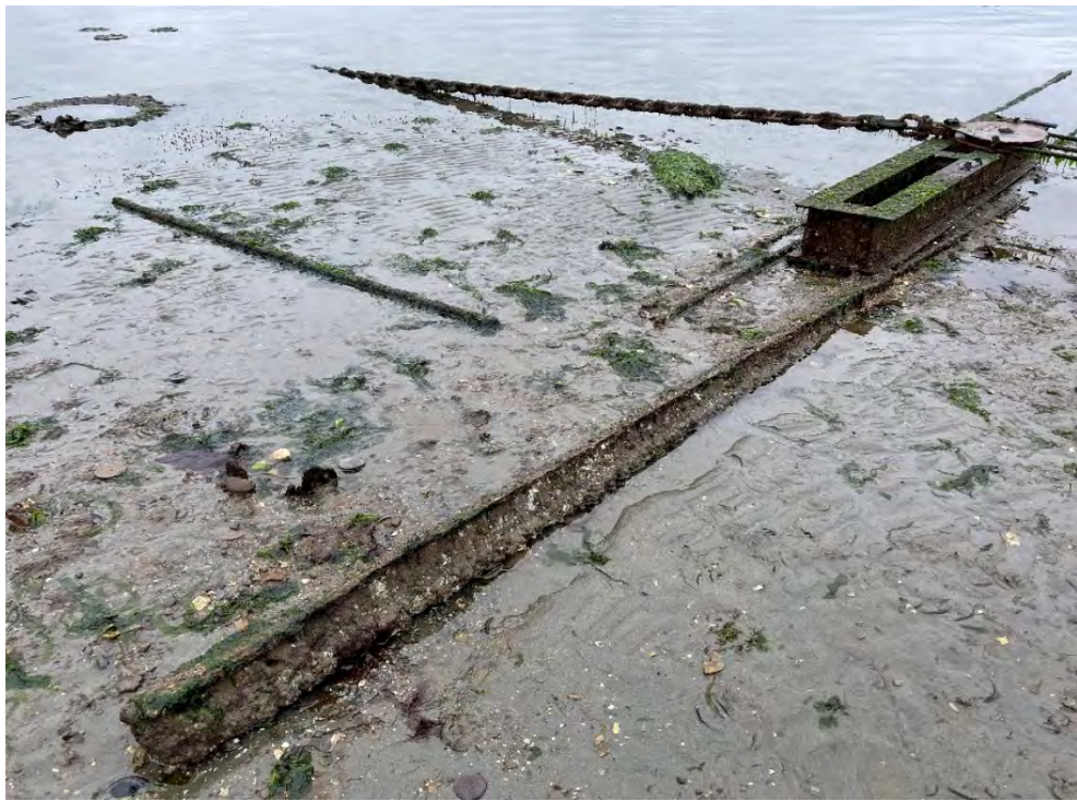
Photo 155: Anchor system at Southern end of track
