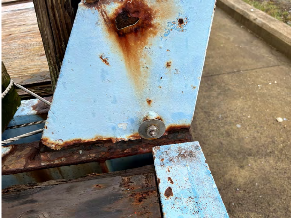
Photo 194: Base of column on cradle
