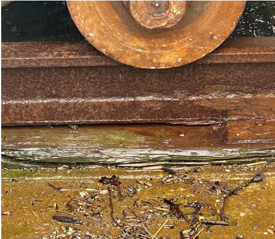
Photo 135: Rail and timber rail North of bulkhead
