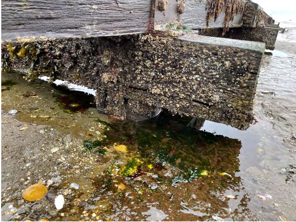
Photo 152: Pile 8B, early stages of hollowing
