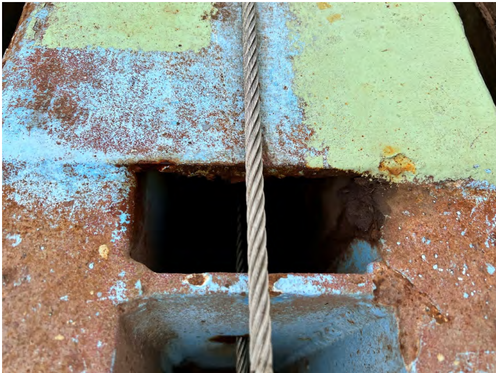
Photo 195: Bilge block wire rope
