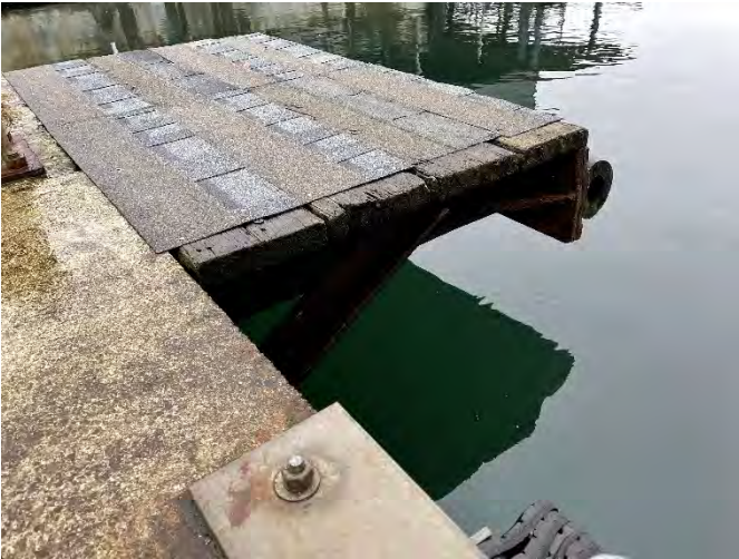
Photo 61: Balcony loading platform
