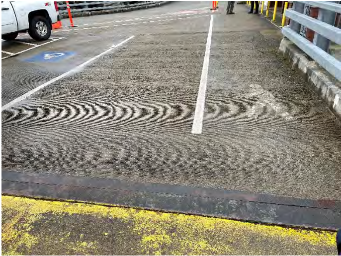
Photo 18: Steel sliding plate
