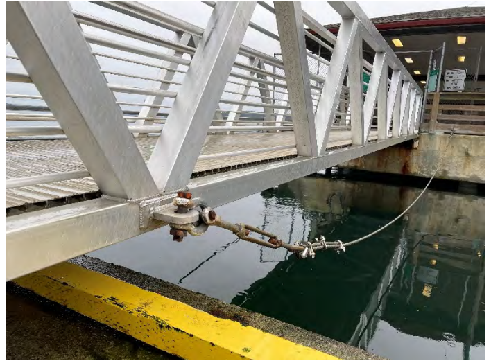
Photo 44: Tie back cable attachment
