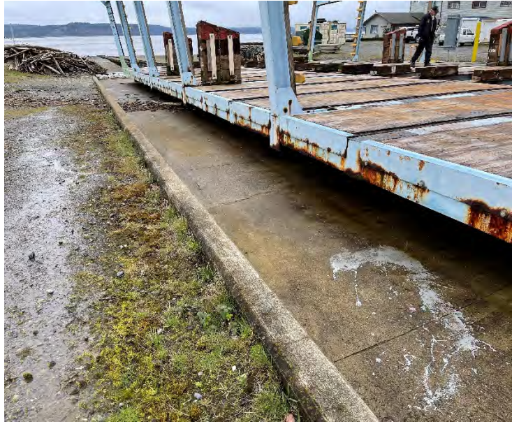
Photo 134: Cradle and concrete North of bulkhead
