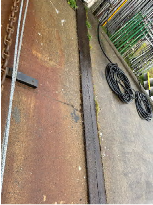
Photo 128: Timber rail beam (A) North of bulkhead
