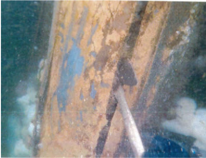
Photo 43: SP1-A holed through
