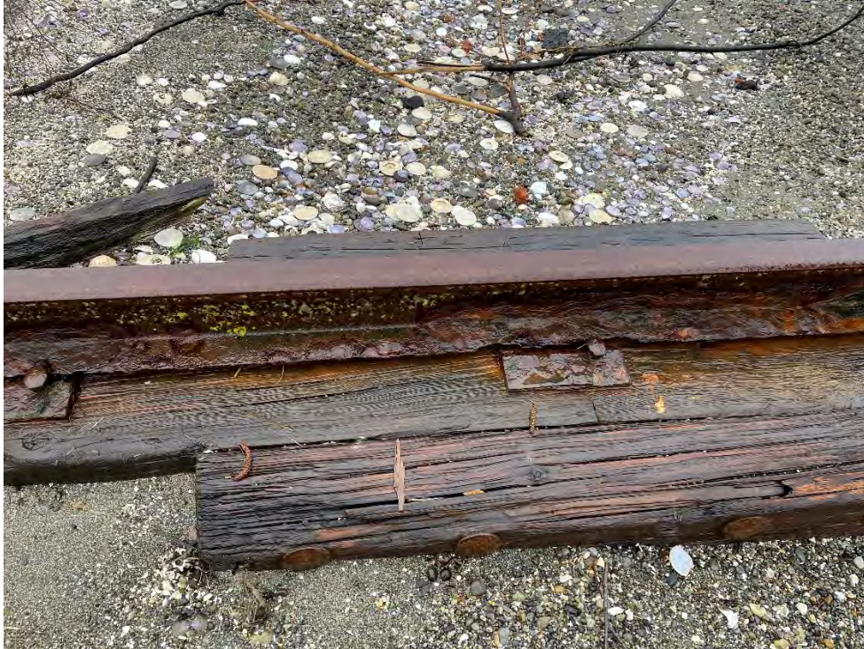
Photo 136: Rail (A) and timber rail South of bulkhead
