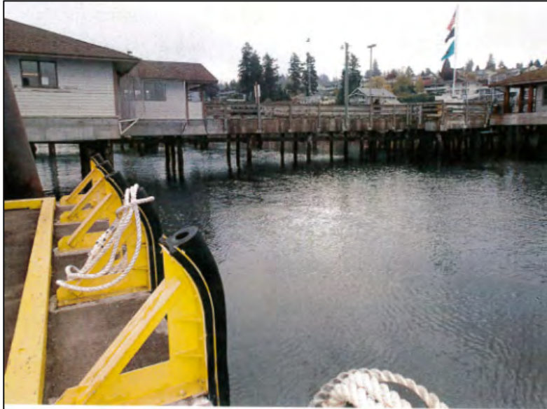
Photo 1B: Steilacoom building trestle
