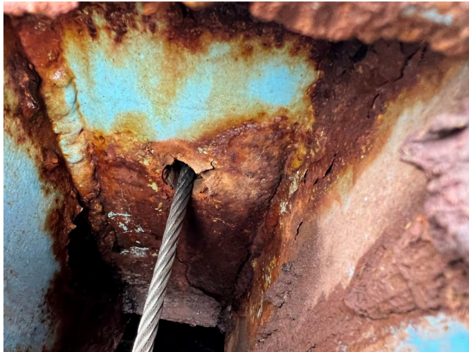
Photo 193: Bilge block wire rope
