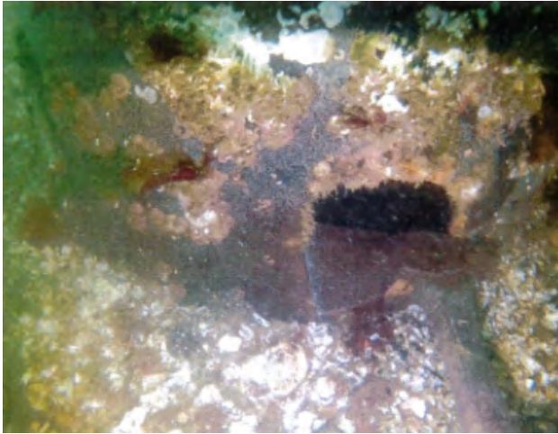
Photo 35: SP1-D holed through
