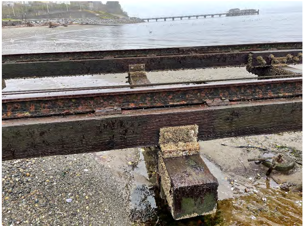
Photo 139: 10 th pile cap from bulkhead
