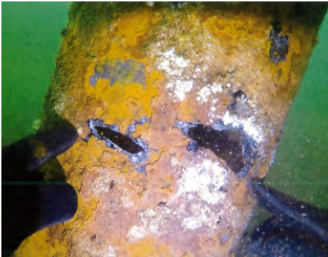
Photo 116: Pile E, 4.5" W x 1.5" H hole and 3.5" W x 0.75" H hole
