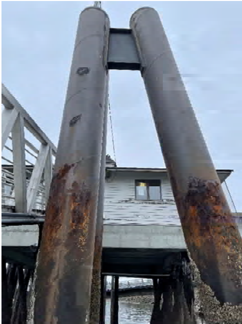
Photo 29: Plumb pile and batter pile
