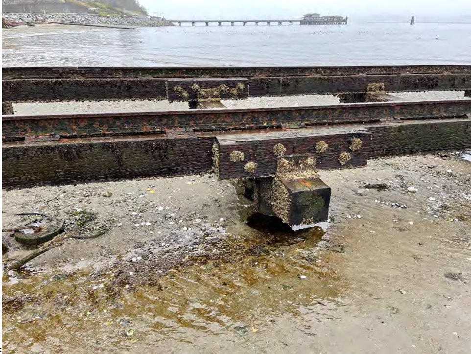
Photo 140: 11 th pile cap from bulkhead
