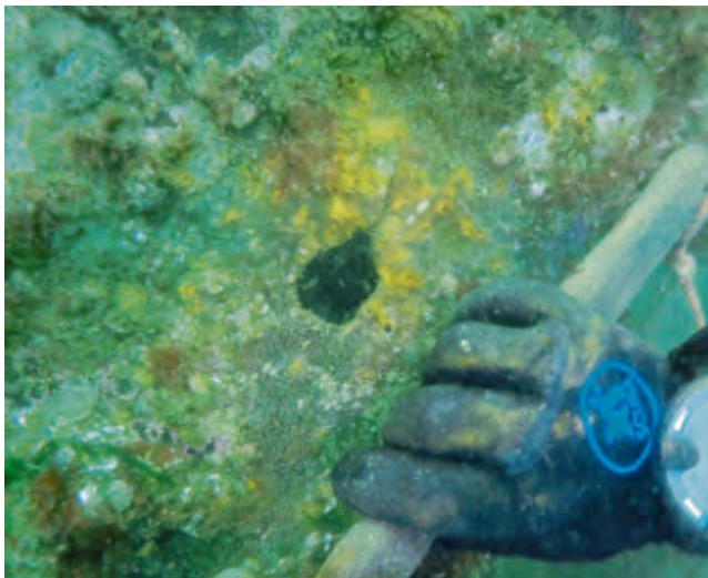
Photo 37: SP3-B holed through
