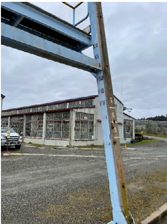
Photo 160: Cradle column at North end
